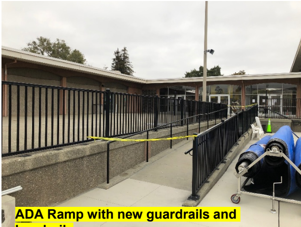
New 42" guardrails and 60" fence
