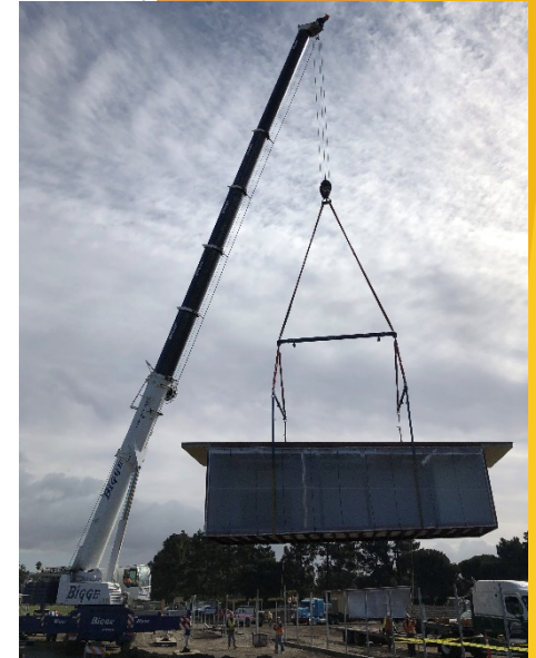
Installing the new Team Room into place
