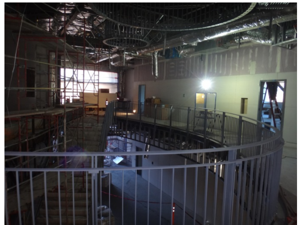
Lobby Stairs at Second Floor
