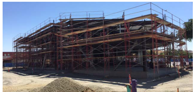
Southwest building view
