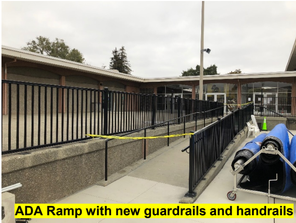
New 42" guardrails and 60" fence
