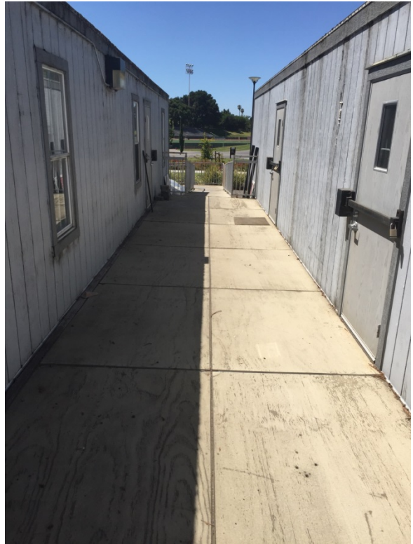
Decking between existing buildings facing ramp
